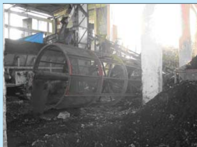
Broken screen at a compost plant
