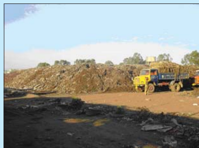
An excessively overloaded compost plant causing odor nuisance and facing resistance from community
